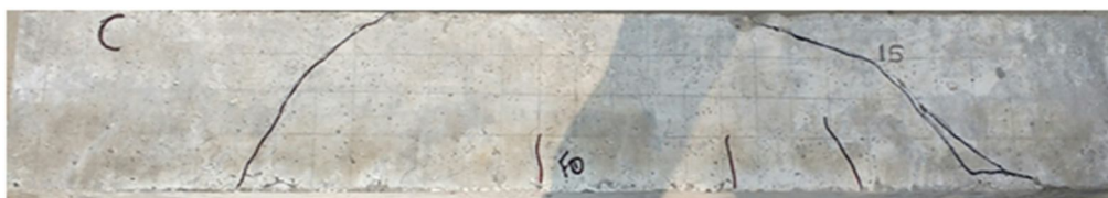
Fig.5 Control beam (C) after Testing
